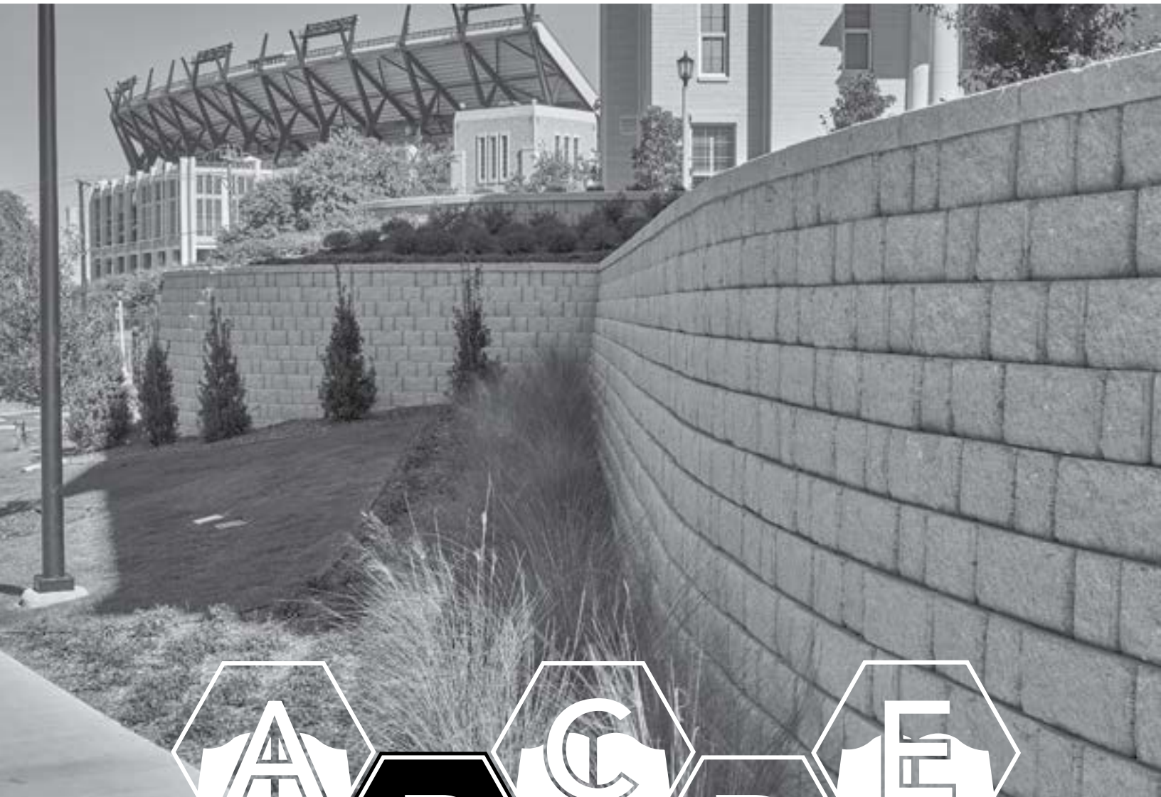
TCU Parking Garage, Fort Worth, Texas; Regal Stone Pro® RockFace 3-pc
