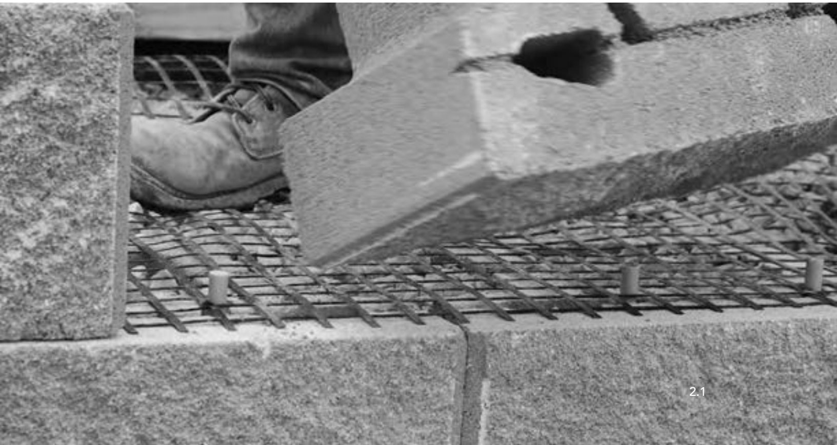
Wall construction with geogrid reinforcement.
